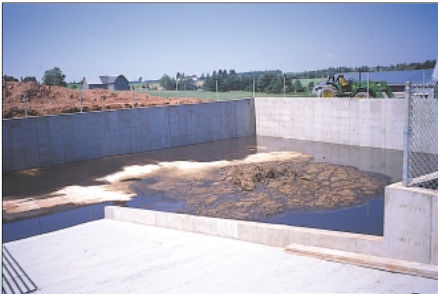
Curbed concrete manure storage with safety fence.
