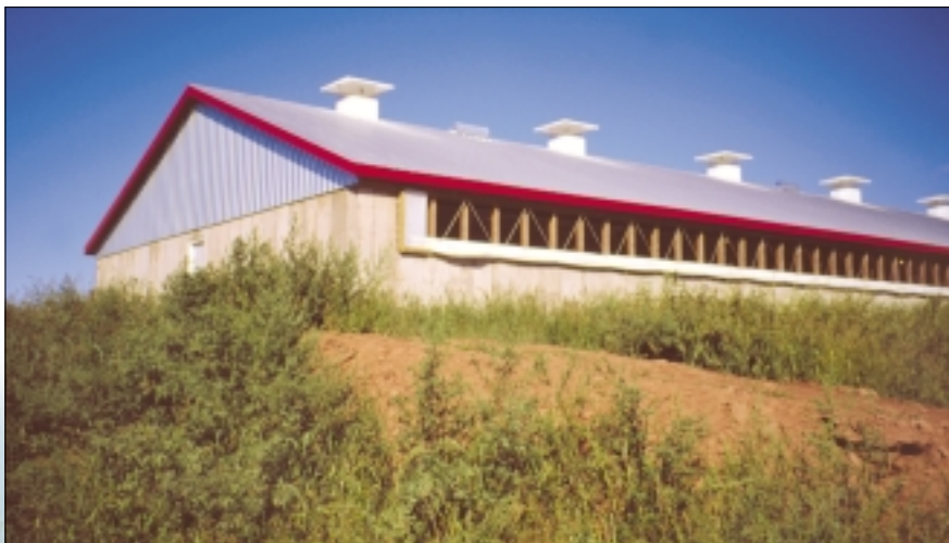
Roof exhaust outlets to maximize air dilution.
