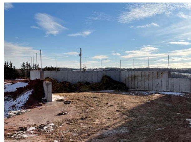
Solid Manure Storage with Push Wall
