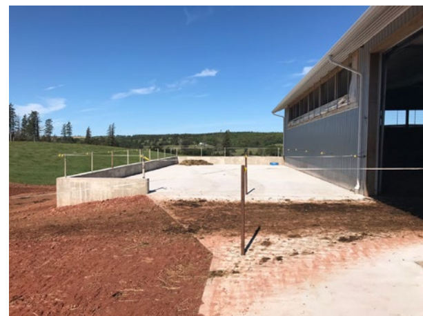
Solid Manure Storage with Curb
