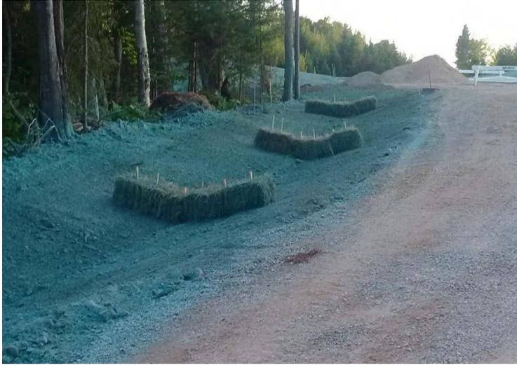
**HAY/STRAW BALES** are a short-term measure often used as check dams. Their use must be limited to ditches with drainage areas less than 0.8 hectares. They must be keyed into the ditch and staked with two stakes angled towards the adjacent bale. Hay/straw bales are best suited as a type of silt fence if they are bound with wire or string. They are
