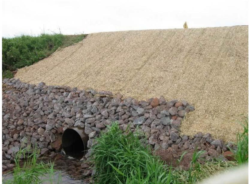
(large surface area of strands) and contains such small openings that it can be used alone as a blanket. Since these materials will decompose over time, they should be used in permanent conveyance channels with the realization that the system's resistance to erosion is based on the type of vegetation planted and the existing soils characteristics.
