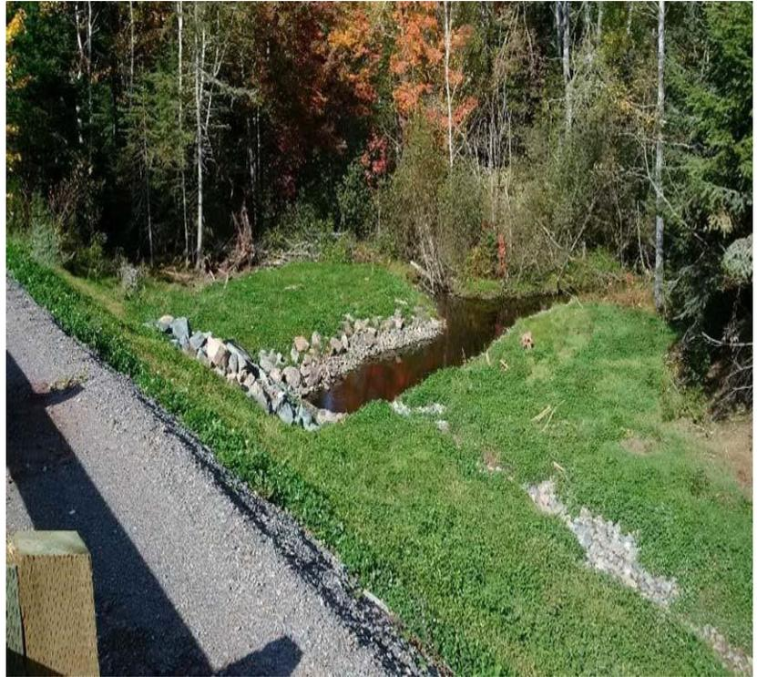
plans. Steep slopes can be seeded but may require fabric mats, pinned to the ground for seeding to work. Temporary stabilization can be achieved by the use of hay mulch or by the use of anti-erosion mats. Seeding is recommended for long term stabilization of exposed slopes.
