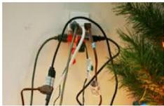
Only use lights and extension cords that are in good condition. Check for frayed wires, bare spots, gaps in the insulation, broken or cracked sockets/plugs, excessive kinking or wear. Check the cords to see if they feel warm when they have been on for a while. If you find any of these signs, replace with an approved Canadian Standards Association (CSA) product.
