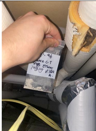
Parging cement on pipe fittings of fiberglass pipe
