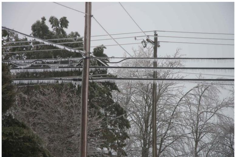
Figure 40. Freezing rain on powerlines. Photo provided by DE Jardine.
