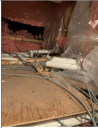
Fiber Glass insulation above ceiling in boiler room.
